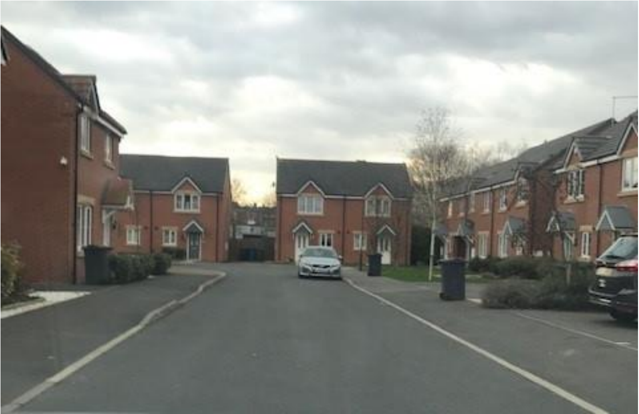
Figure AM-A6: On street parking occurring on carriageway width of 5.5 metres
