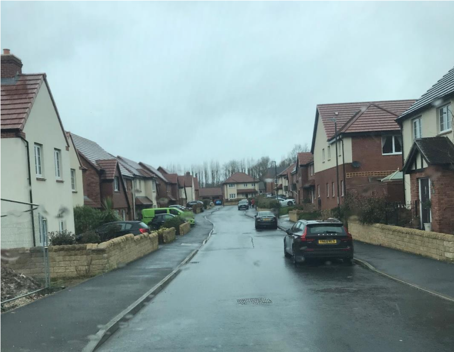
Figure AM-A4: On-street parking occurring on carriageway width of 5.5 metres
