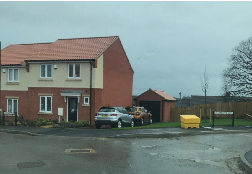
Figure AM-A1: Utilisation of triple tandem parking at Dunston Lane, Chesterfield CHE/16/00016/OUT Housebuilder: William Davis
